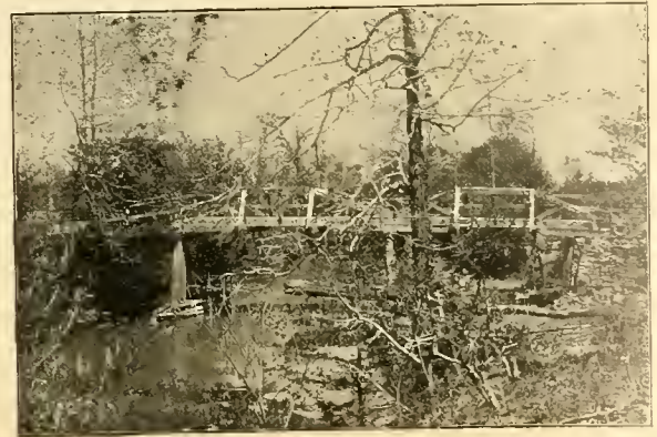
Reed's Bridge, National Military Park.
